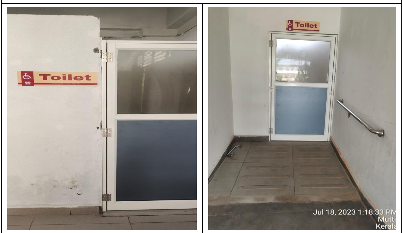
Fig-8: Toilet Facilities
